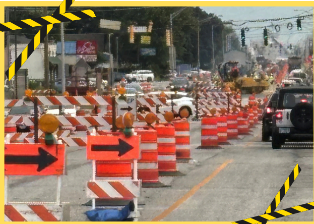
55th St. looking east at the La Grange Rd. intersection.
